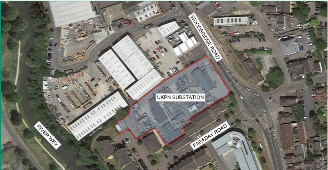
Figure 4-1: UKPN Primary Substation Location (Google Maps, © 2022 Google)
